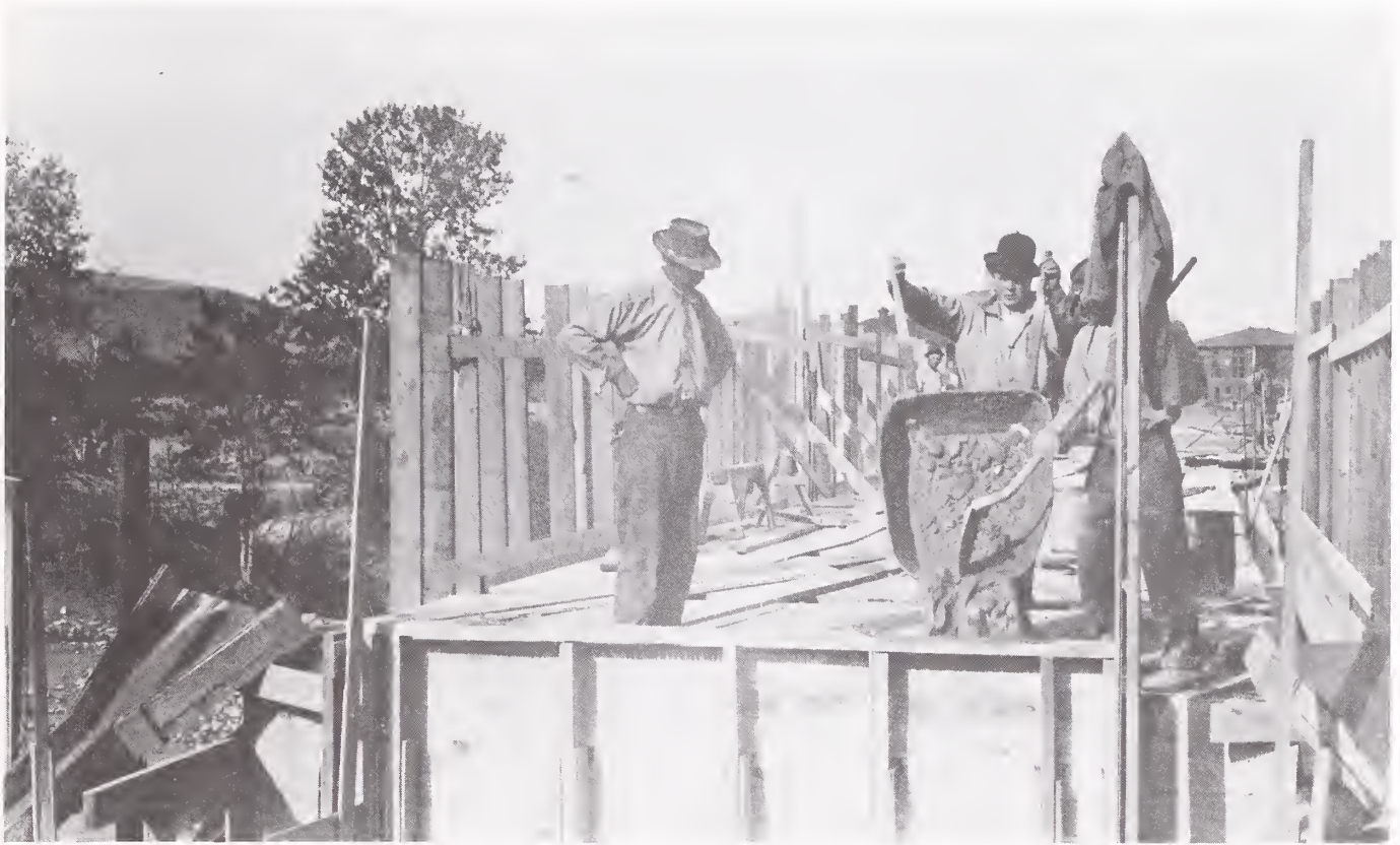
Pouring the concrete into the forms. This method was used until at least World War II (Montana Historical Society).
